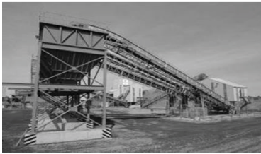
Fig. 2: Metal Recovery Plant.
