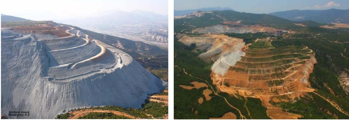
Fig 2: View of the restoration works of the deposition (Prefecture of Kozani 2012)
